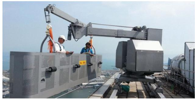
**Access for Maintenance:** A building maintenance unit (BMU) allows safe, easy access for maintenance crews; it obviates riskier and more labour-intensive methods, such as scaffolding.
